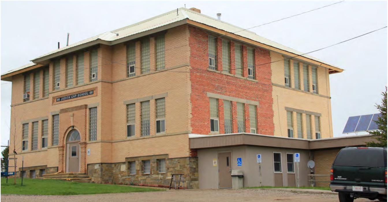
Figure 3: The 1911 Judith Gap schoolhouse, with hipped roof extended from a flat roof, showing the modification to the roofing associated with extending the building to the rear. Photograph courtesy of Carroll Van West.
